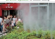
saving, outdoor cooling system with Semi-Dry Fog®, which provides effective evaporative cooling effect without wetting people.
